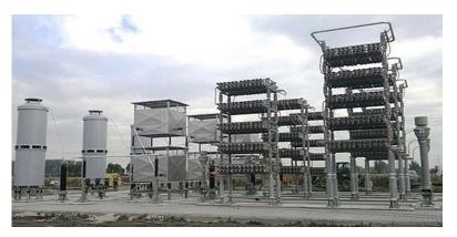
Figure 3: To master the high voltage of 250 kV to 300 kV phase-to-ground in accordance with the regulations, frames are developed for the capacitors, upon which each horizontal assembly is installed using individual capacitors. These frames are separated electrically using insulators and assembled at the customer site to form a tower 7 m to 10 m high. A total of 30 to 45 frames are required depending on the power of the plant.
